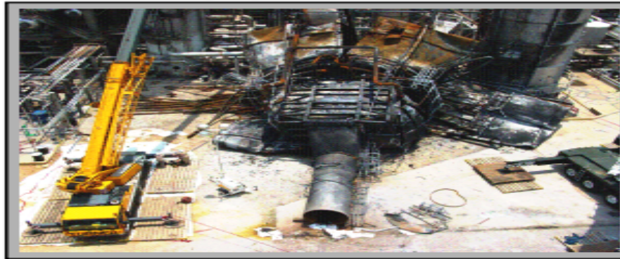
Photograph of the heater and adjacent column
